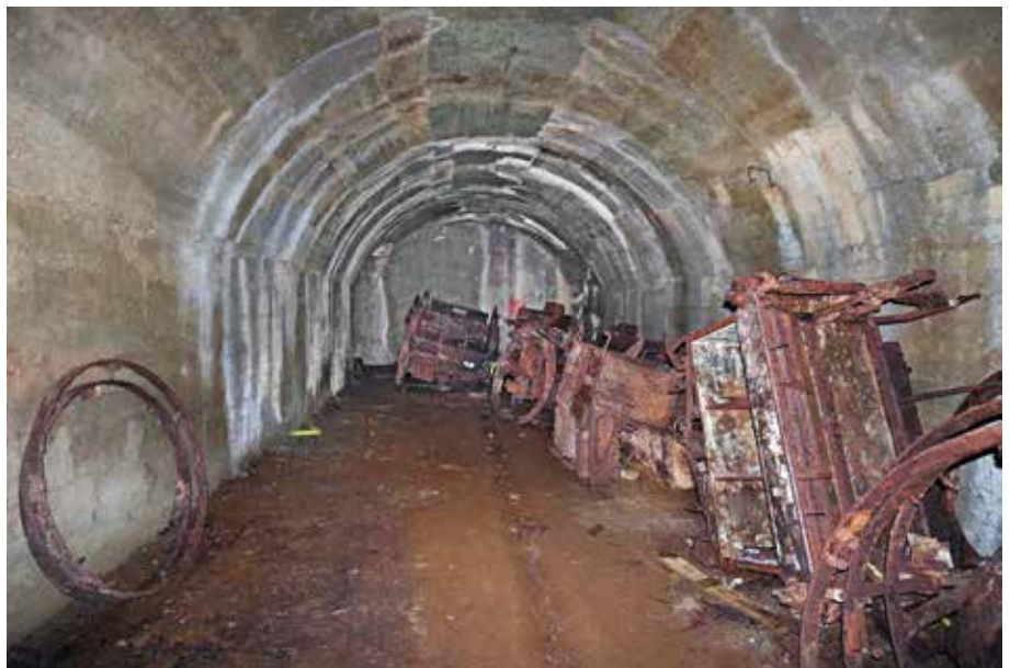
Two of the remaining three lined storage chambers still contain rusting German equipment. Gun limbers now without their wooden wheels which have rotted away and field kitchens are seen here
